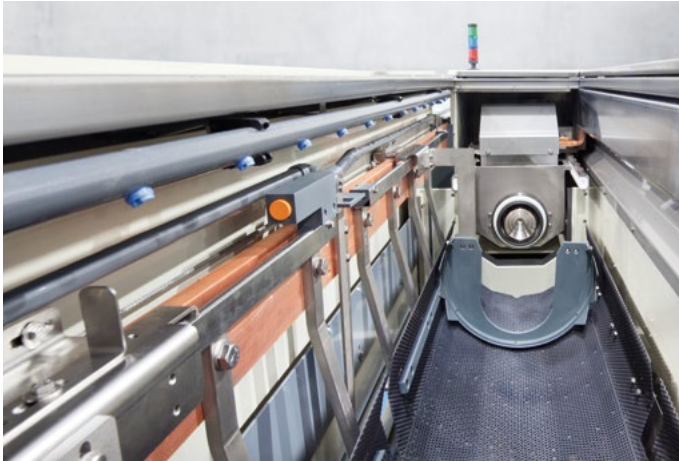
Copper tank, view of anode basket Kupferbad, Blick in den Anodenkorb
